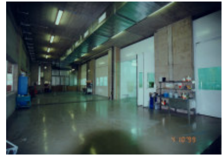
Netstal Maschinen AG, painting area, 540 m 2 , electrical conductive VIBALIT 3E AS epoxy floor topping
