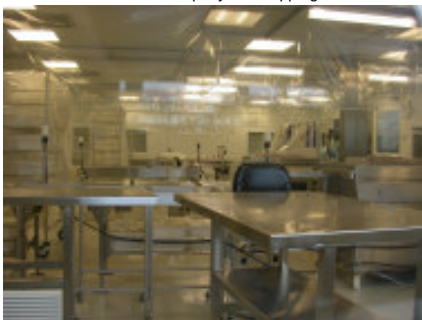
Sulzer Orthopedics Winterthur, clean rooms 610 m 2 , electric conductive VIBALIT 3E AS epoxy floor topping
