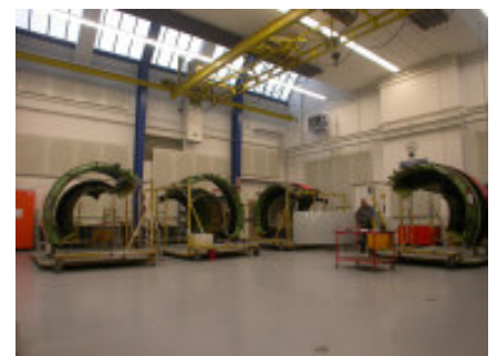
SR Technics, airplane engine service plant, VIBALIT 3E NS, Non-skid floor topping, 640 m 2 . Applied on 8 days old concrete
