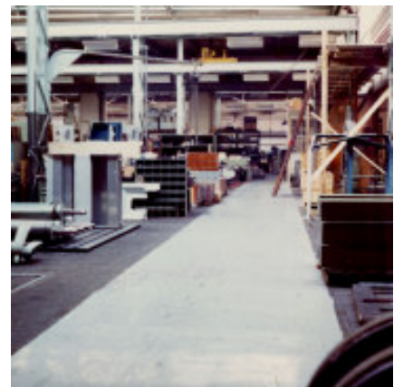
VIBALIT 3E industrial floor topping in traffic area, Bühler AG Uzwil
