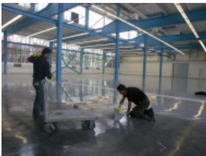
Application of VIBALIT 3E epoxy floor topping at Sulzer Immobilien Rüti, manufacturing plant 2'300 m 2
