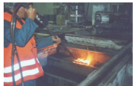
Swiss railway depot Chiasso, flame blasting to clean the concrete and remove from oil and grease
