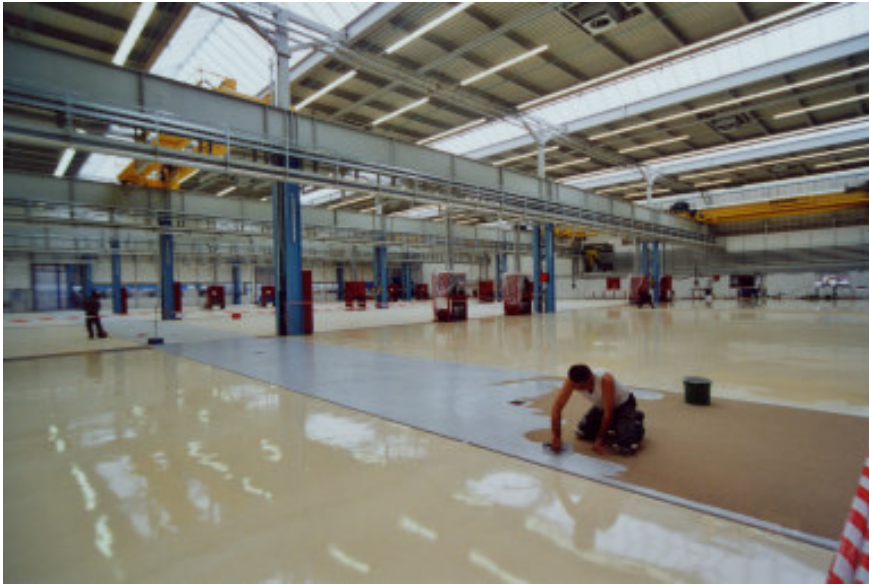
Netstal Maschinen AG, Manufacturing plant 6'735 m 2 , machine assembling area with VIBALIT 3E, traffic area with VIBALIT 3E NS non-skid epoxy floor toppings
