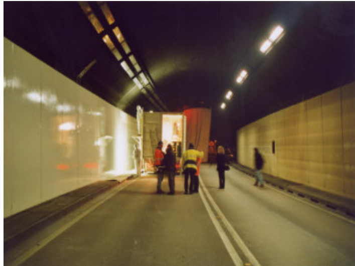
City Tunnel Bregenz, 8200 m 2
